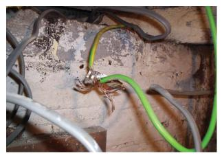
Absence of a reliable means of earthing
