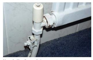
Unmarked bonding conductor
