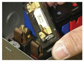
Checking a fuse carrier (base missing)
