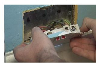
Socket-outlet with broken face plate
