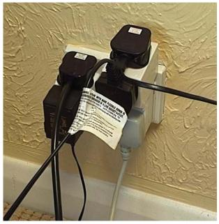
A potentially overloaded socket-outlet
