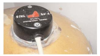
Older immersion heater without thermal cut-out
