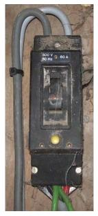
60 A voltage-operated earth-leakage circuit-breaker. (Photo courtesy of RF Lighting)
