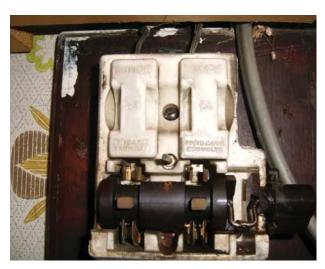
Double-pole switch with fuses in each pole
