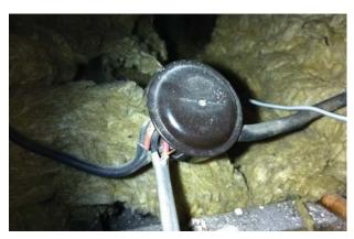
Cable sheaths not taken inside non-conducting enclosure
